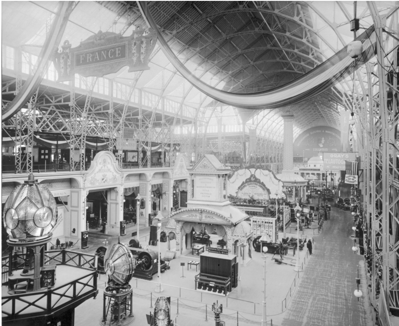
Interior view of Electricity Building, 1893 World's Fair.
